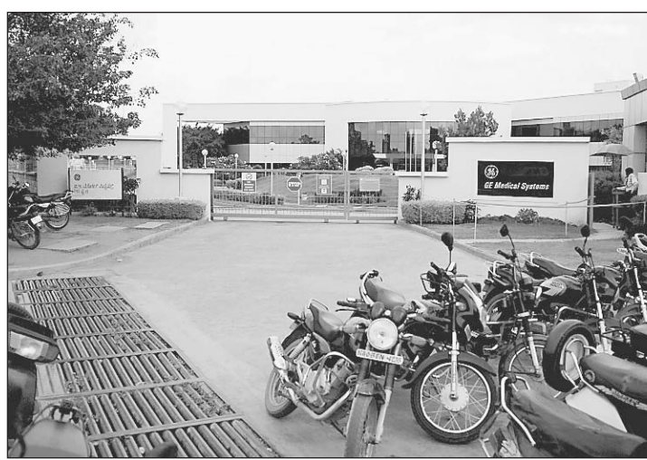
General Electric's offices are located in the Whitefields suburb east of Bangalore, India. The firm has teamed up with Wipro Ltd. to distribute low-cost ultrasound machines.
